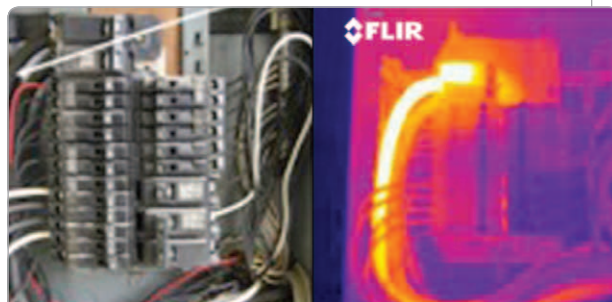
Hot Spot in an Electrical Panel
